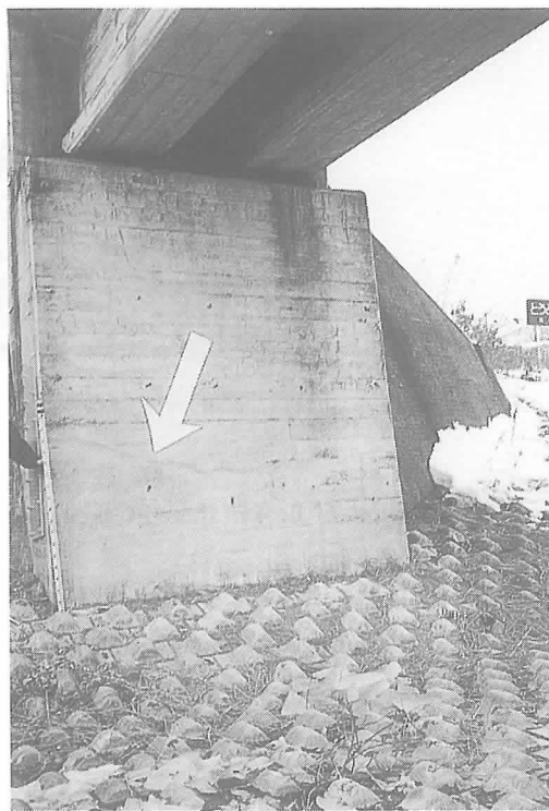
Photo-3 Crack at 50 cm above reinforcing steel girder, between Chokubetsu steel section decreases point on and Atsunai abutment (T-beam of RC, between Ikeda and Shoei)
