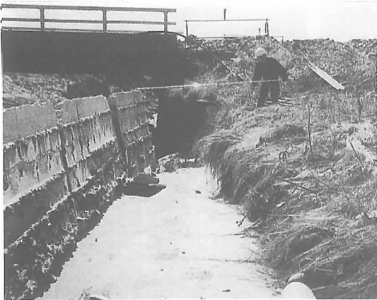
Photo-7 Moving and collapsing of retaining wall due to retreating tsunami (concrete retaining wall, Matsumae in Okushiri)
