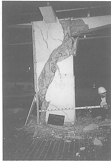
Photo-22 Concrete destroyed, broken stirrups, deformation and yield of longitudinal steel at recessed steel section past of RC pier (the first floor of 3-story high school building in Hachinohe city)
