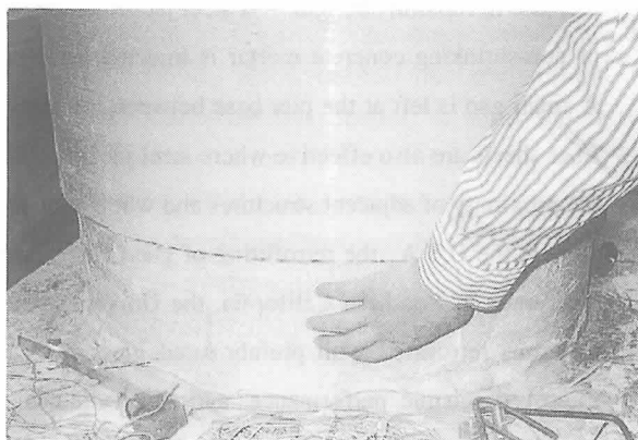
Photo-31 Retrofitting the part between the pier and base to retain original structural design
