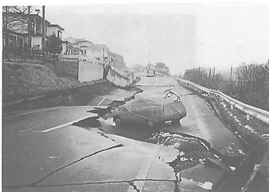
Photo-23 Collapse of a road embankment subbase caused an L-shaped concrete retaining wall to slide 3.5 m and subside by 2.5 m (at Matsugaoka in Hachinohe city)
