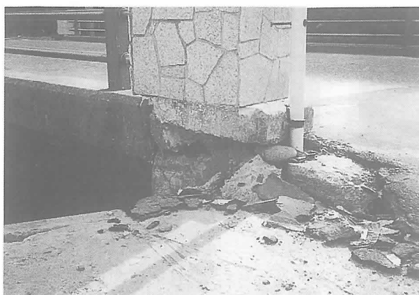
Photo-13 Broken concrete of abutment (concrete girder bridge, Okushiri in Okushiri town)
