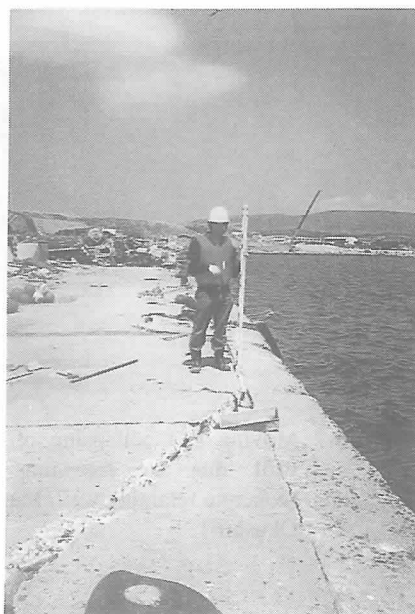
Photo-12 Crack and breaking on lighter's wharf by subsidence (concrete apron, Aonae in Okushiri)
