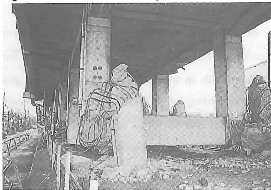
Photo-25 Concrete destroyed, stirrups failed and the longitudinal reinforcing steel yielded and deformed at recessed part of RC pier (express railway bridge, PC girder, near Mukogawa river in Nishinomiya city)
