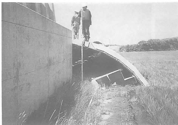
Photo-11 The collapsed snow shelter base wall of arch and the collapsed arch (PC arch structure Senjyozaka in Okushiri, just before completion in July 1993)
