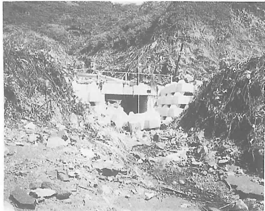
Photo-8 Damage to parapet and abutment (concrete girder bridge, Monai in Okushiri)
