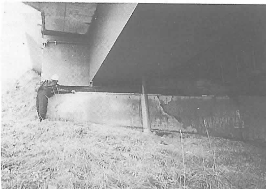
Photo-18 Failure of the anchor support, cracking, and scaling of the concrete abutment. The width of the abutment: 275 cm at the upper part and 460 cm at the lower part. (road bridge, 3 spans continuous, 2 main girders box section, Midorimachi in Nakashibetsu town)
