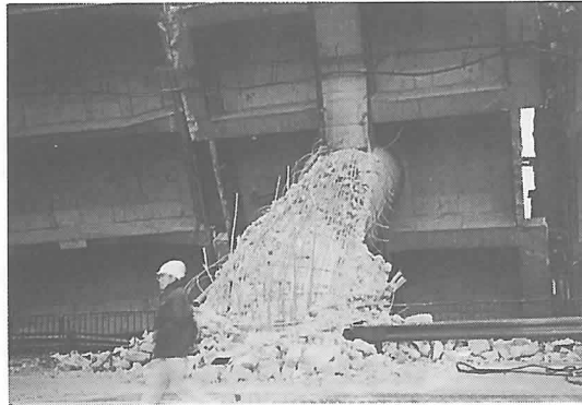
Photo-24 Expressway piers and girders failed and collapsed (PC bridge constructed in 1969, at Fukae Bonjyochyo, Higashinada Ward in Kobe city)
