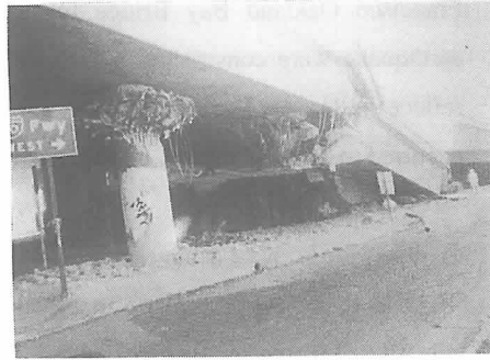
Photo-28 Damaged bridge piers - the cores completely disintegrated at I-10 during the Northridge earthquake.
