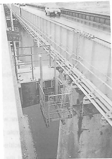
Photo-21 Concrete pier of steel girder bridge tilted and damaged a part of concrete pier of pedestrian bridge by crashing onto each other (road bridge: constructed in 1931, pedestrian bridge: enlarge a construction in 1972. Kumanodou – Naganawa-shironai Funawatasi in Hachinohe city)
