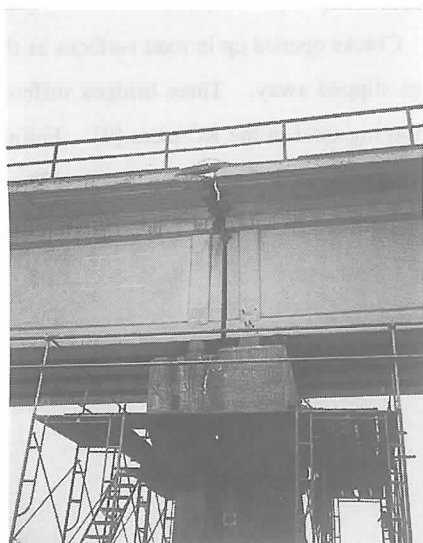
Photo-4 Broken shoe and concrete girder bridge (PCT: T beam of prestressed concrete bridge, between Hobetsu and Ikeda)
