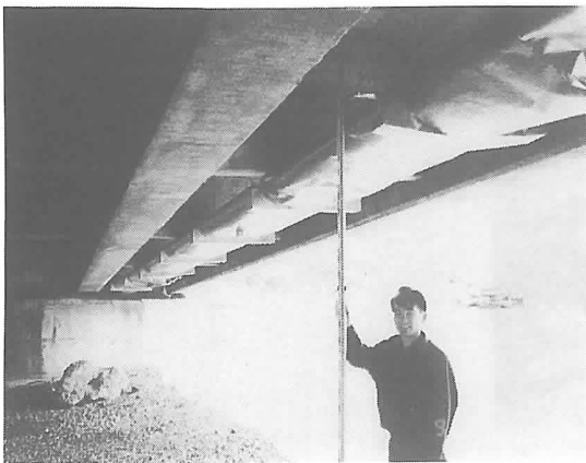
Photo-9 Deformation of steel plate covers of water supply pipe underneath caused by tsunami (concrete girder bridge, Shimamaki)
