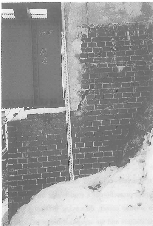
Photo-2 Crack and inclination of abutment
