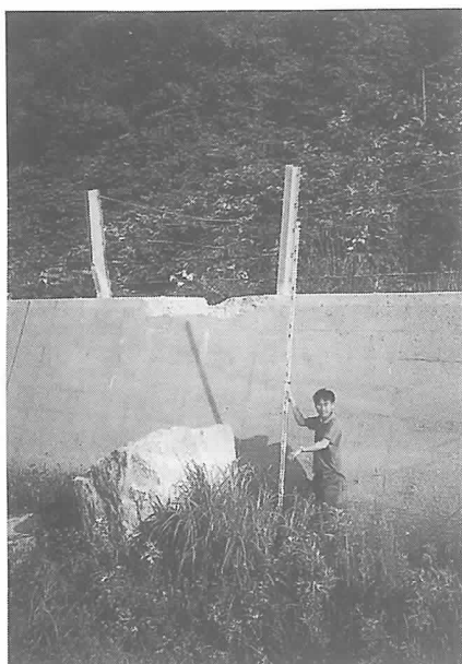
Photo-14 Falling stones caused by earthquake and damage to retaining wall (concrete retaining wall, Shimamaki)
