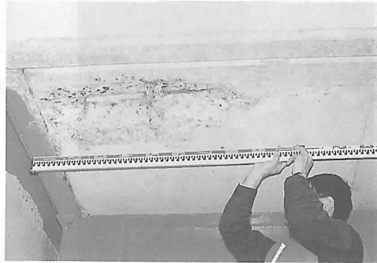
Photo-17 Failure and scaling of concrete, exposure of stirrup steel, and other damage were caused when the girder was crushed against the abutment (road bridge, composite girder, Furen in Bekkai town)
