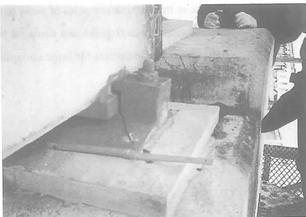
Photo-5 Broken side stopper of shoe (PC girder bridge, between Ineshi and Makubetsu)
