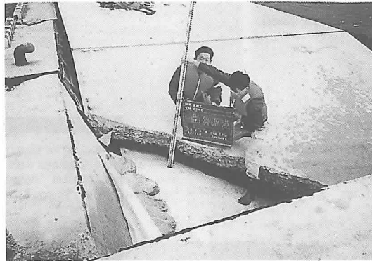
Photo-20 Wharf tilted and sank and broke the concrete plate of apron (fishing port, Habomai in Nemuro city)
