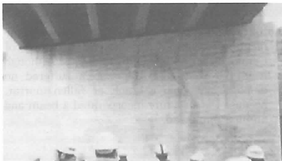
Photograph 41 Bridge abutment damaged by crustal deformation from volcanic activity along the Doou Expressway.
