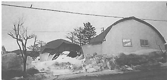
Photograph 1 An agricultural warehouse in the Kitami district that collapsed under a heavy load of snow in January, 2004. (Saroma-cho Sakae, along National Highway Route 333)
