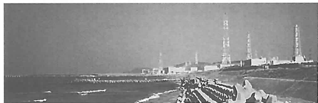
Photograph 33 After the earthquake, the Kashiwazaki nuclear power plants were able to quickly resume normal operations because the plants were designed using dynamic analysis and adequate measures had been taken to prevent liquefaction and other earthquake related problem.
