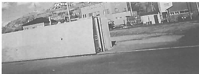
Photograph 37 The basic functions of the embankment gate of the anti tidal wave quay in Hanasaki port, Nemuro City were not damaged by the Kushiro Oki Earthquake (29th November in 2004), but were damaged by the Hokkaido Toho Oki Earthquake in 1994. An aftershock (December 7, 2004) of the Kushiro Oki Earthquake also did no damage to the gate but only because heavy snow protected it according to one report.
