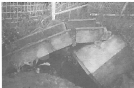
Photograph 40 Road drain damaged by crustal deformation from volcanic activity.
