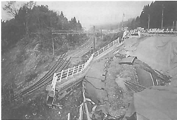
Photograph 29 The collapsed cliff beside National Road Route 17 and the JR Joetsu Line.
