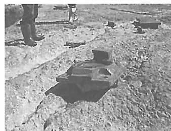
Photographs 6, 7 The support beam attachment points and the destroyed support beams of the bridge.
