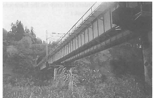
Photograph 15 This plate girder bridge on the JR Joetsu Line is in fairly good condition, but a bolt securing a railroad tie fell out.
