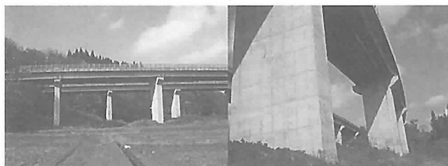
Photographs 21, 22 The piers of the Kanetsu Expressway are in fairly good condition.
