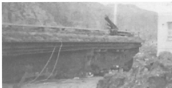
Photograph 43 RC-beam for road bridge on route 230, washed away by a mudflow.
