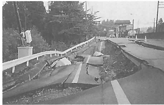
Photograph 31 Sections of the prefecture regional road route in Ojiya City collapsed and suffered extensive damage to the pavement, sub-base, course, and sub-grade.
