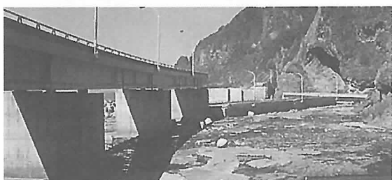
Photograph 3 The broken girders and piers of Omori Bridge (completed October, 1985) on National Road Route 229. (The piers between 4 spans and the girders fell only on the Kamoenai side, to the southeast.)
