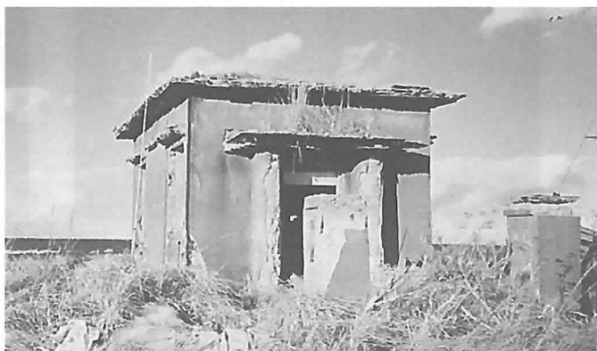
Photograph 38 The Northern Territories communications system of the former Department of Communications is a cultural asset. Although it is 100 years old, the system suffered no damage, not even a crack or fallen mortar, because the structure incorporated a beam and an inner bulkhead.
