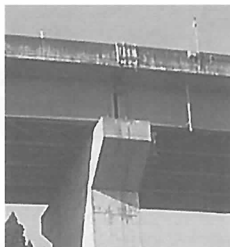
Photograph 23 The concrete edges of these girders were only slightly damaged in the earthquake.
