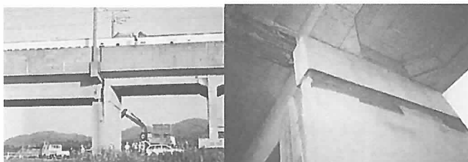
Photographs 25, 26 The concrete scaling at plumb down of the reverse side of the bridge abutment was scraped at the derailment site (Photograph at left). The center of the upper part of the RC pier on Higashi-oh-shin-e Bridge in the same site (photographed from the west side). It blows concrete into the shave part which drops scaling be in scrape (November 7-8, 2004).
