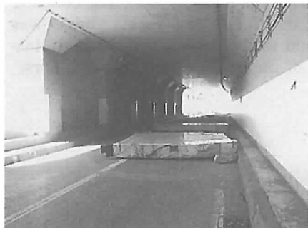
Photograph 2 This concrete shelter wall on National road route 229 in Kamoenai (near Omori Bridge) was toppled by the strong wind and waves generated by Typhoon 18.
