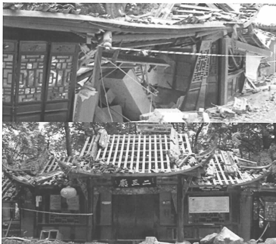
Fig.47. Damage of wooden structure in Dujiangyan
