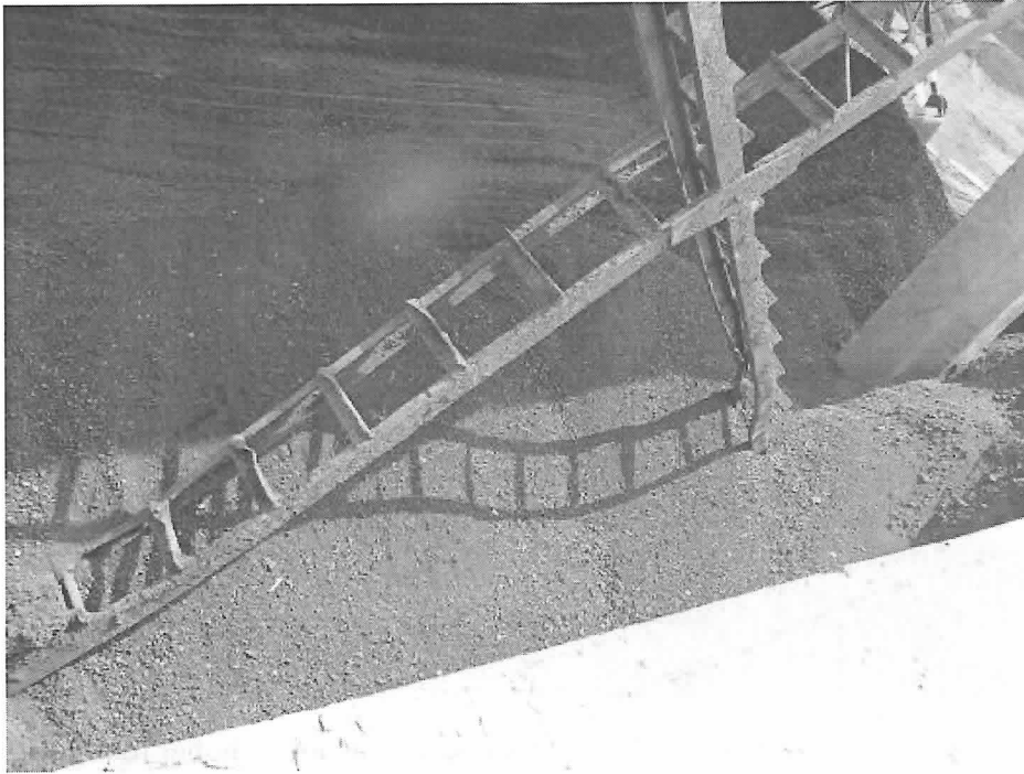
Fig.86. Support bulking between columns of storage of coal factory buildings in a beer company
