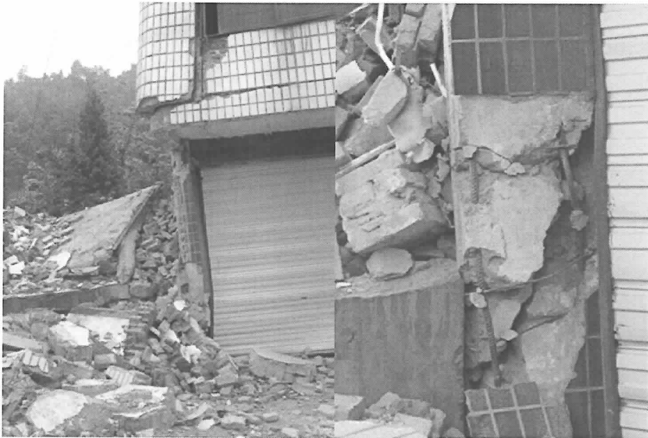
Fig.43. Column damage of frame structure in Jinhua
