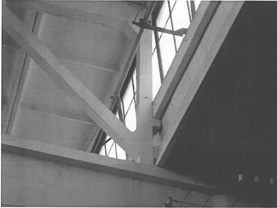
Fig.84. Frame column cracking of sunroof
