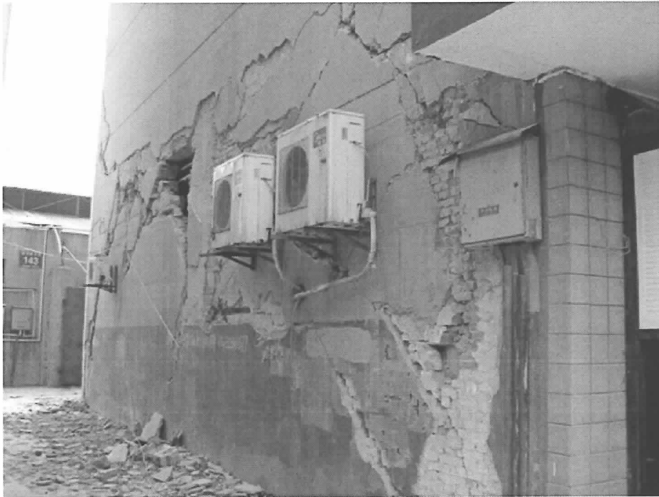
Fig.33. Wall damage in second floor of masonry structure with bottom frame in Mianzhu
