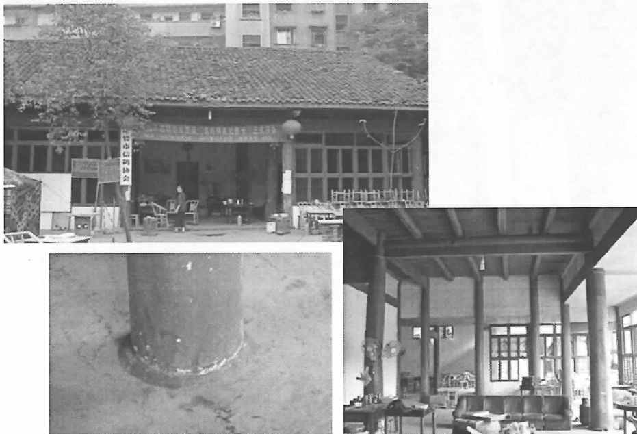
Fig.44. Column displacement of wooden structure in Mianzhu
