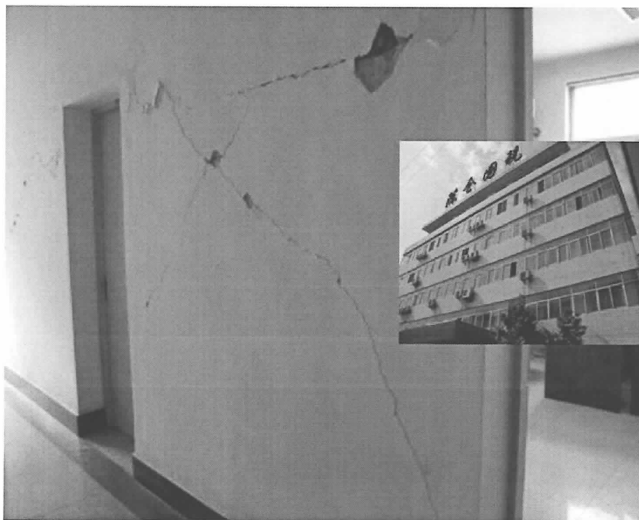
Fig.76. Inner longitudinal wall cracks of an inland revenue department office building
