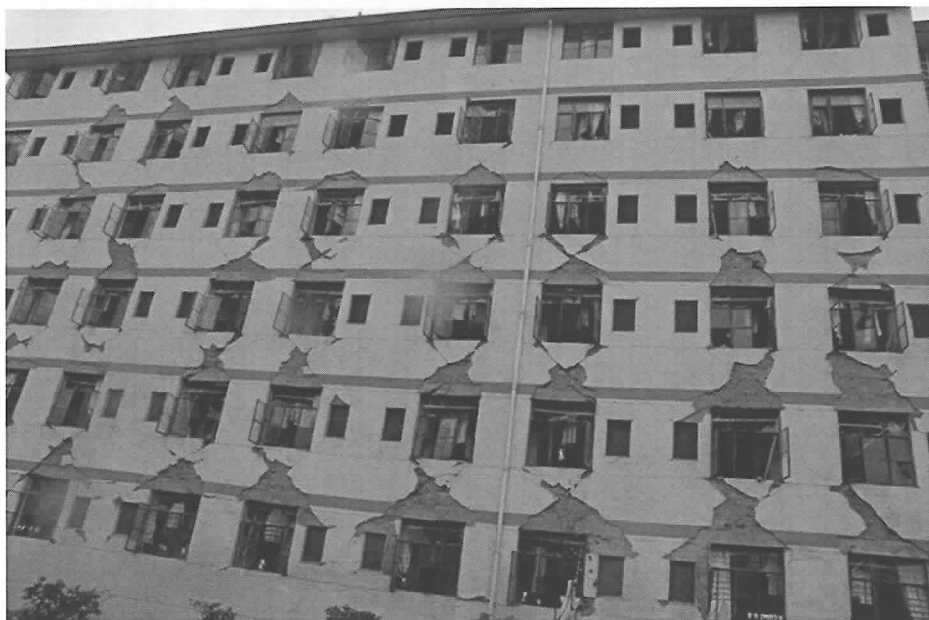
Fig.18. Destruction of masonry structure in Hanwang
