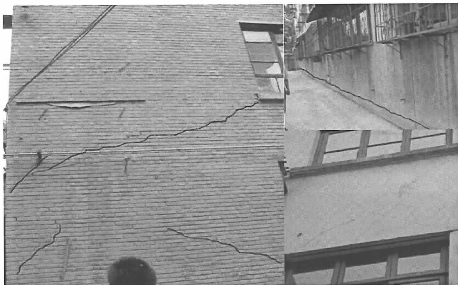
Fig.114. Cracks of brick outer wall
