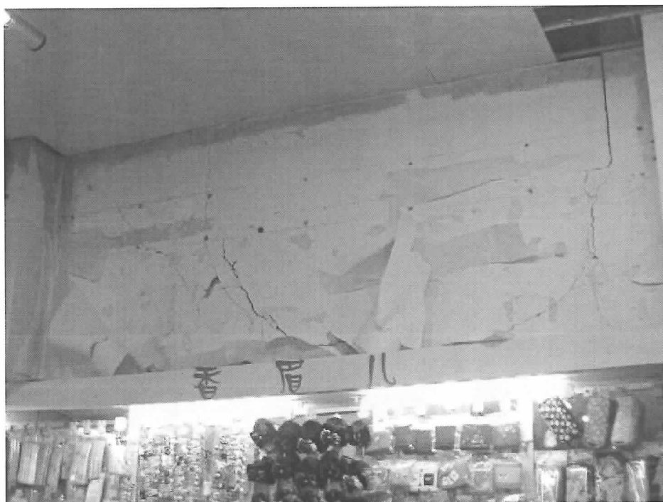
Fig.110. Damage of brick interior wall
