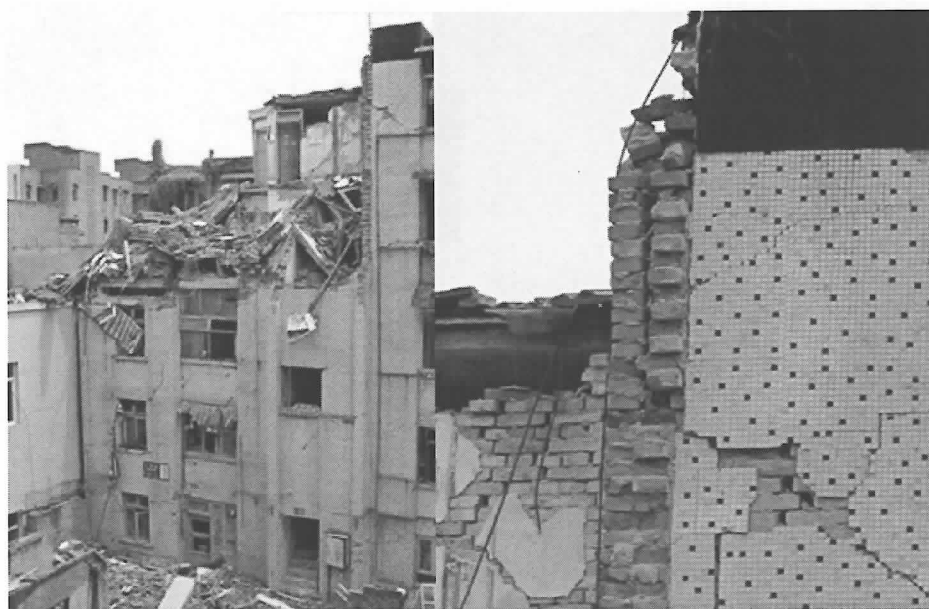
Fig.30. Corner damage caused by the stiffness change of a building in Mianzhu
