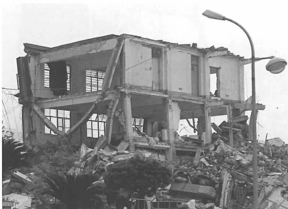
Fig.41. Damage of frame structure in Hanwang
