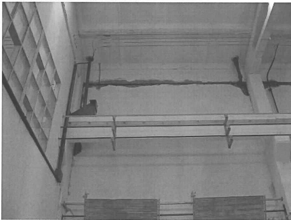
Fig.85. Horizontal crack bottom the beam of longitudinal wall
