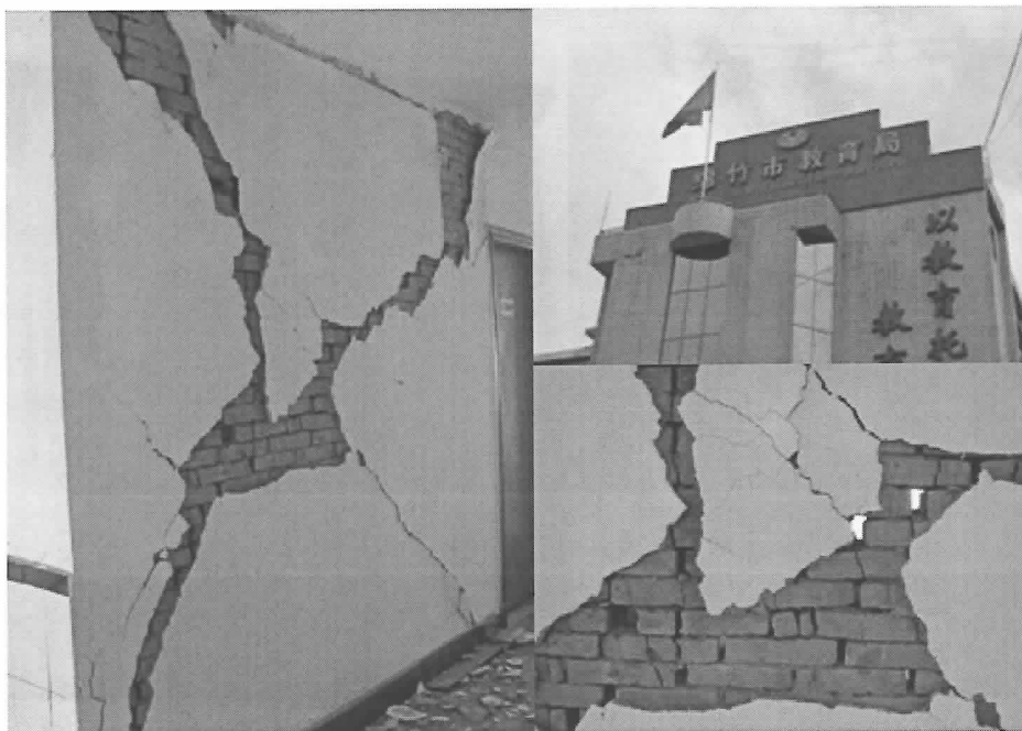
Fig.25. Wall damage of masonry structure in Mianzhu
