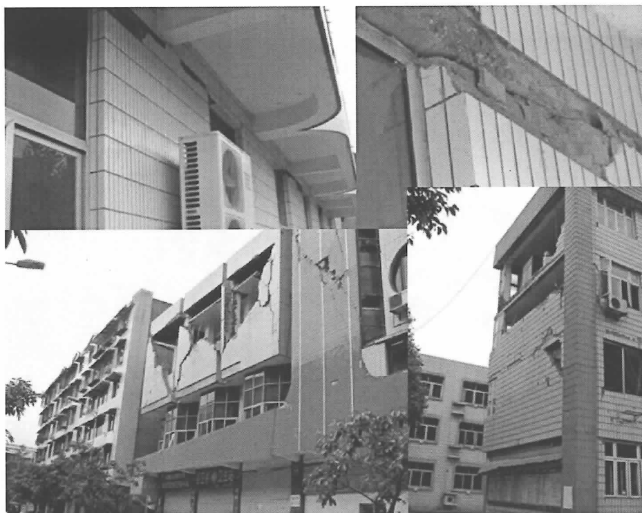
Fig.37. Wall damage of frame structure in Mianzhu
