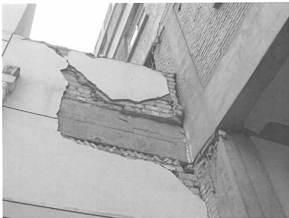
Fig.111. Frame structure damage of a restaurant in Chencang district
