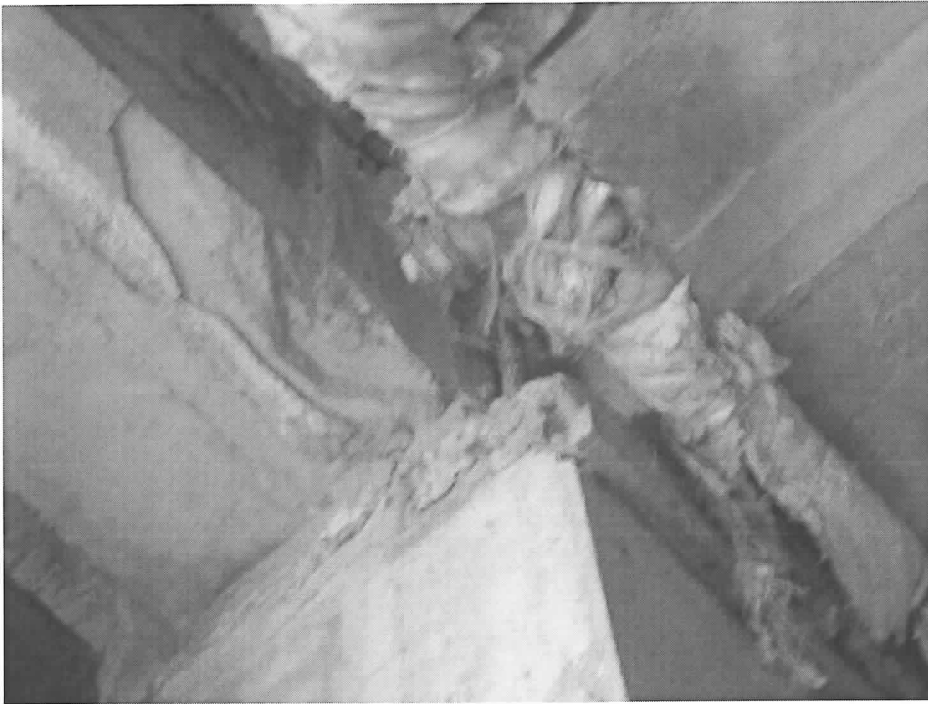
Fig.98. Column yield near node zone, steel drums outside, and has been out of work.
