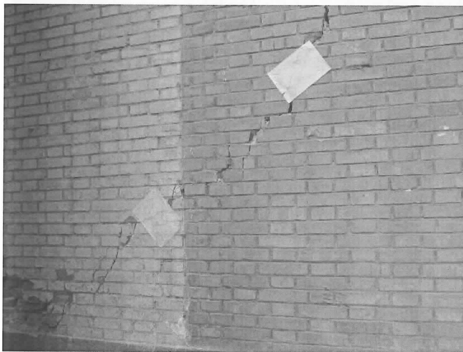
Fig.108. Damage of south outer wall
