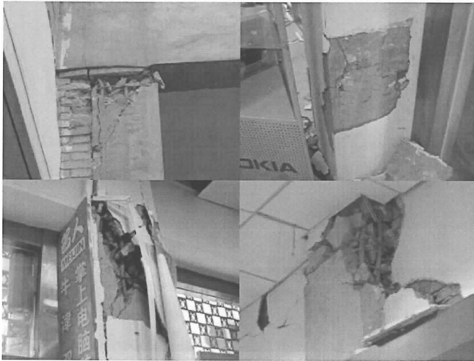
Fig.112. Column damage
