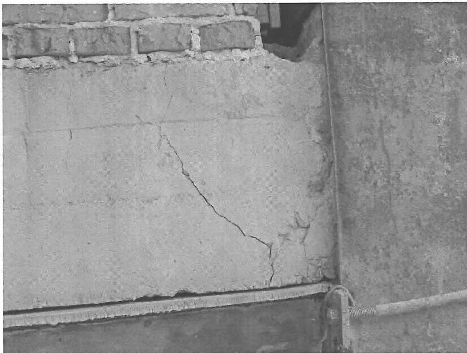
Fig.99. Shear failure at the end of beam
