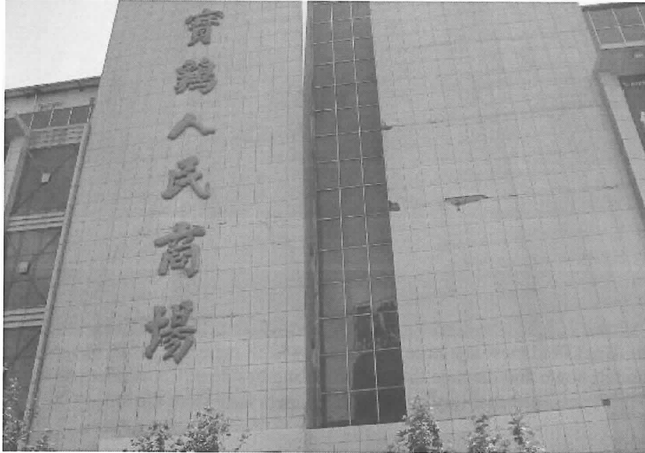
Fig.96. Shopping mall wall decoration damage in Baoji city
