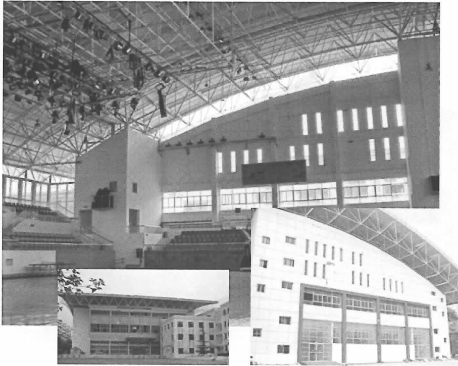
Fig.50. Space truss structure in Hanwang
