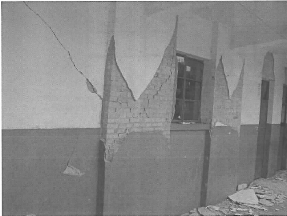
Fig.63. Destruction of brick columns under the beam
