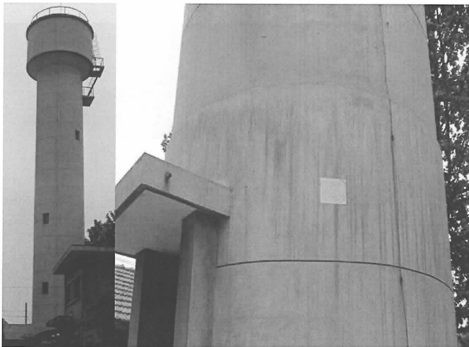
Fig.89. Masonry structure tower is 33 meters high 15 meters circumference, 700mm of wall thickness. There are a number of circular cracks from bottom to top; interval of them is about 3 meters, crack width decrease with height, no vertical cracks.
