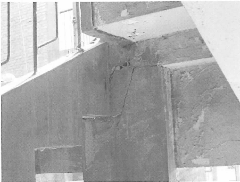
Fig.103. Damage of constructional column
