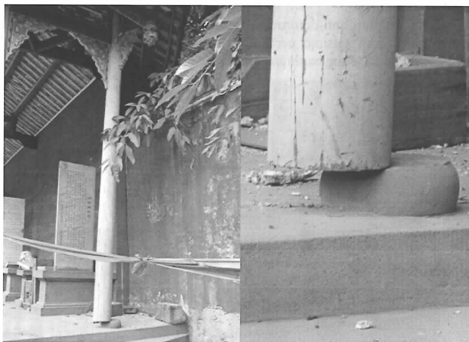
Fig.46. Column displacement of wooden structure in Mianzhu
