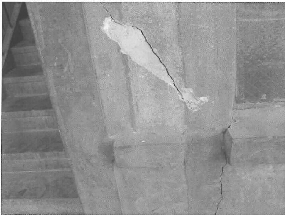
Fig.105. Shear failure at the stair column of the third floor
