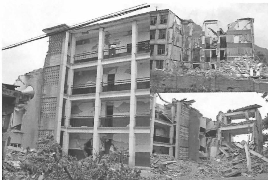
Fig.26. Destruction of masonry structure in Hanwang
