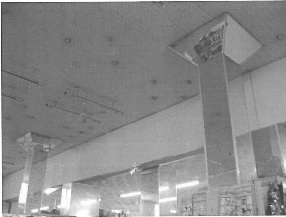
Fig.106. Inner frames and masonry mixed structure of a shopping center in Chencang district
