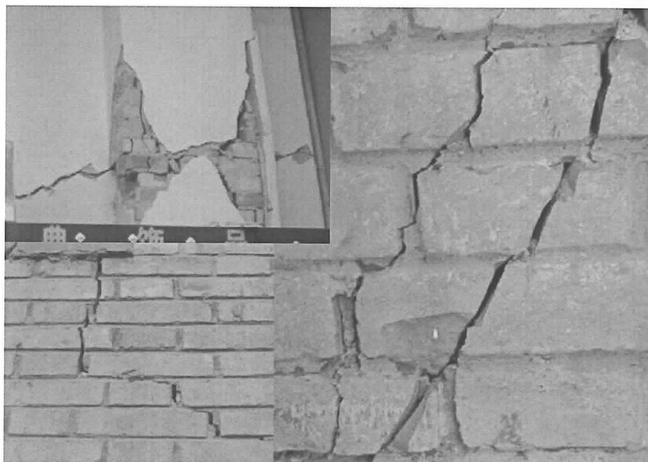
Fig.109. Damage of brick wall and column
