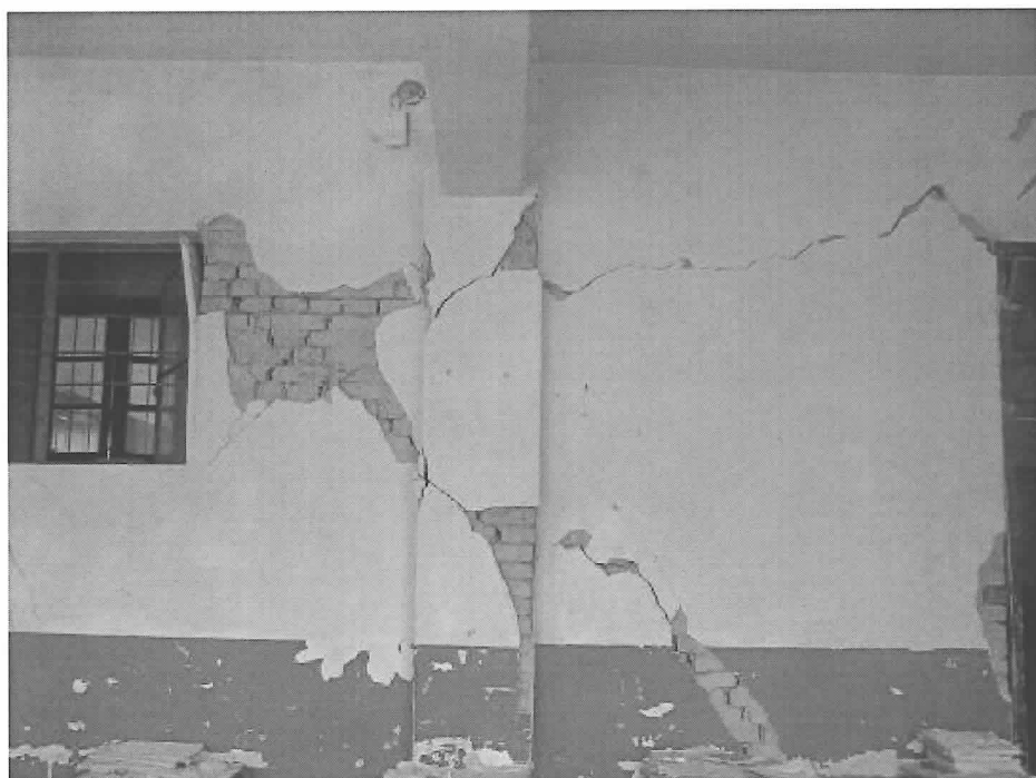
Fig.60. Destruction of brick columns under the beam
