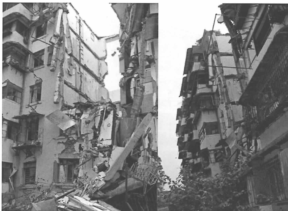
Fig.28. Destruction of masonry structure in Hanwang
