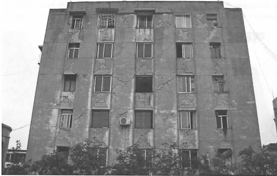
Fig.19. Destruction of masonry structure in Mianzhu
