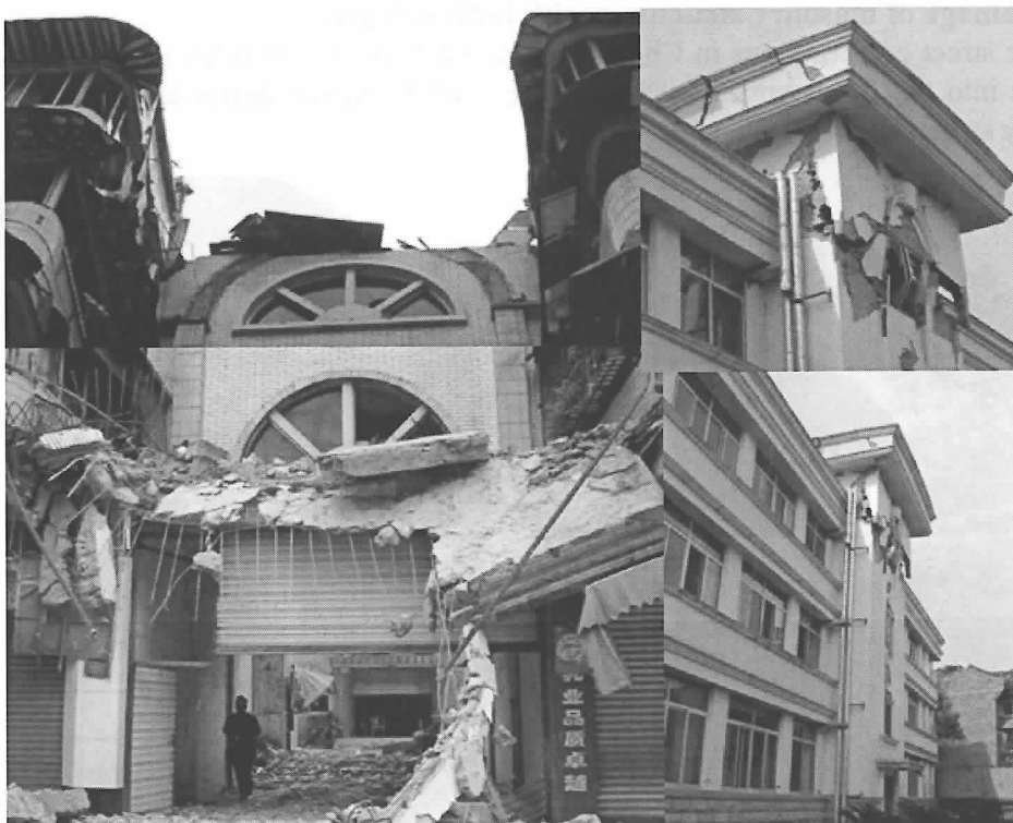
Fig.29. Secondary disaster caused by protruding parapet and staircase damage in Mianzhu
