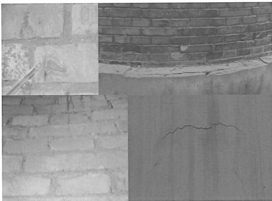
Fig.91. Masonry structure tower with 6 ring beams is 30 meters high, There is one circular cracks at the site of 1 meter from bottom, There are diagonal cracks and vertical cracks between first and second ring beam.
