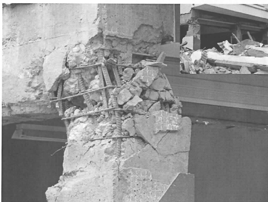
Fig.39. Column damage of frame structure in Hanwang
