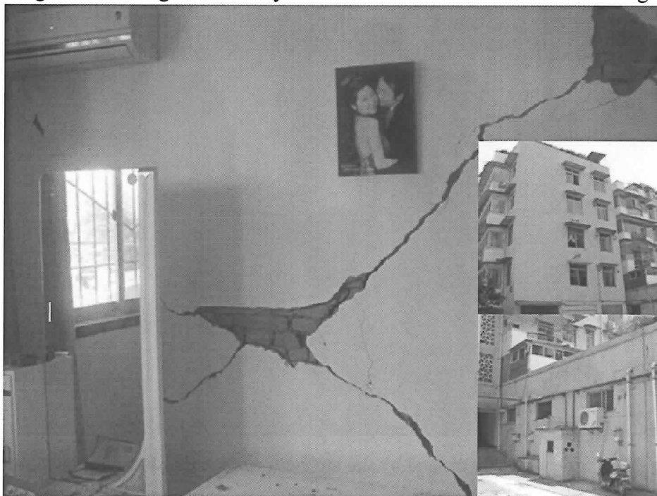
Fig.32. Wall damage in second floor of masonry structure with bottom frame in Mianzhu
