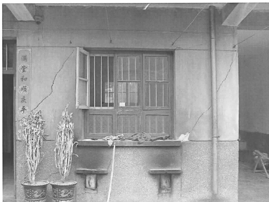
Fig.71. Cracking wall in front of the house
