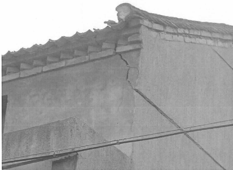
Fig.70. Gable cracks
