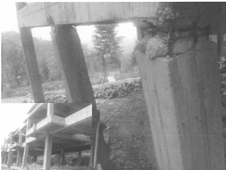
Fig.40. Column damage of frame structure in Jiulong
