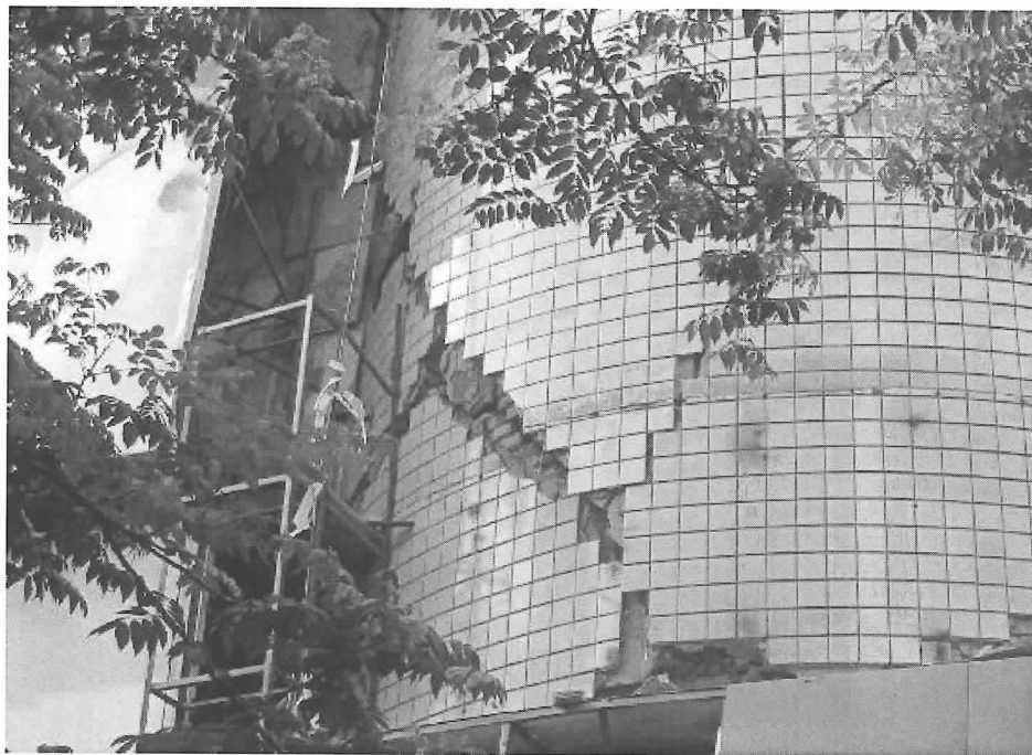
Fig.97. Stair hall arc wall damage of a shop in Chencang district
