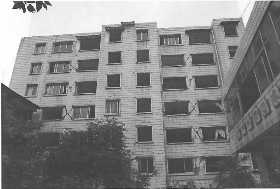
Fig.17. Destruction of masonry structure in Hanwang
