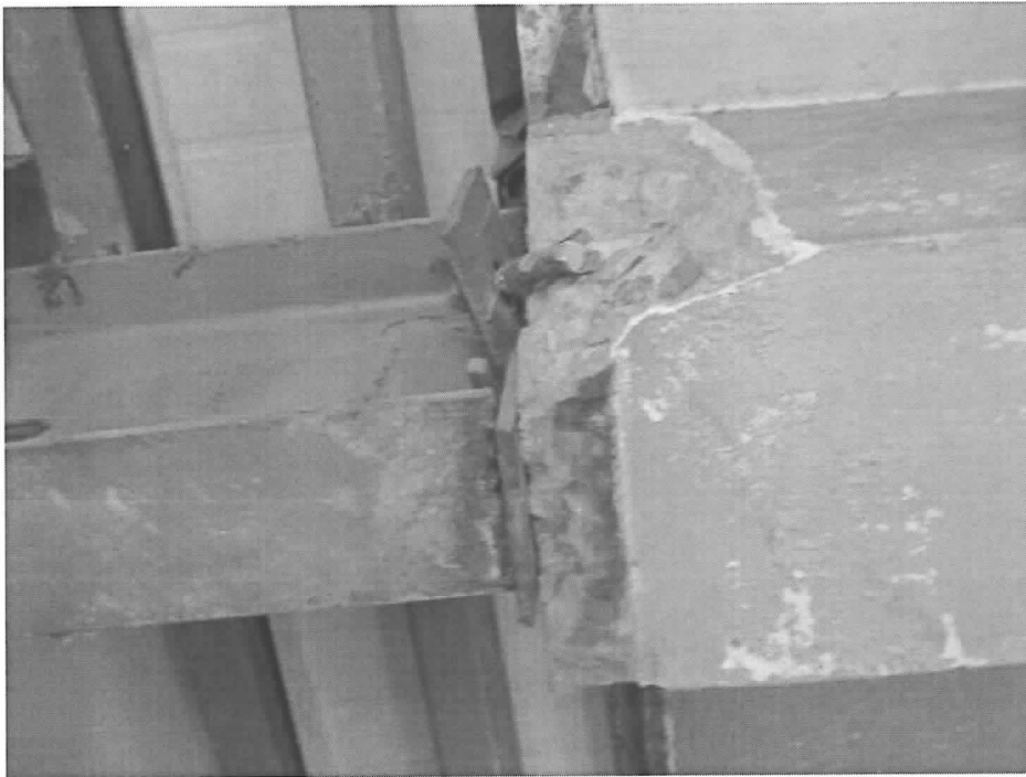
Fig.102. Snap broken at the connection between steel beam and RC beam
