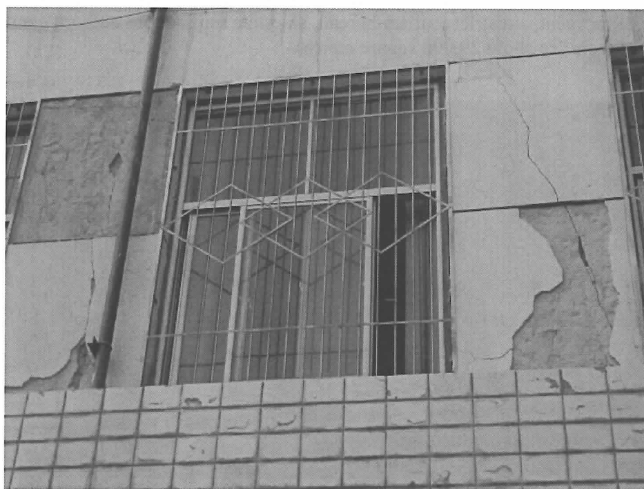
Fig.77. Exterior wall cracks of a district tourism bureau office building
