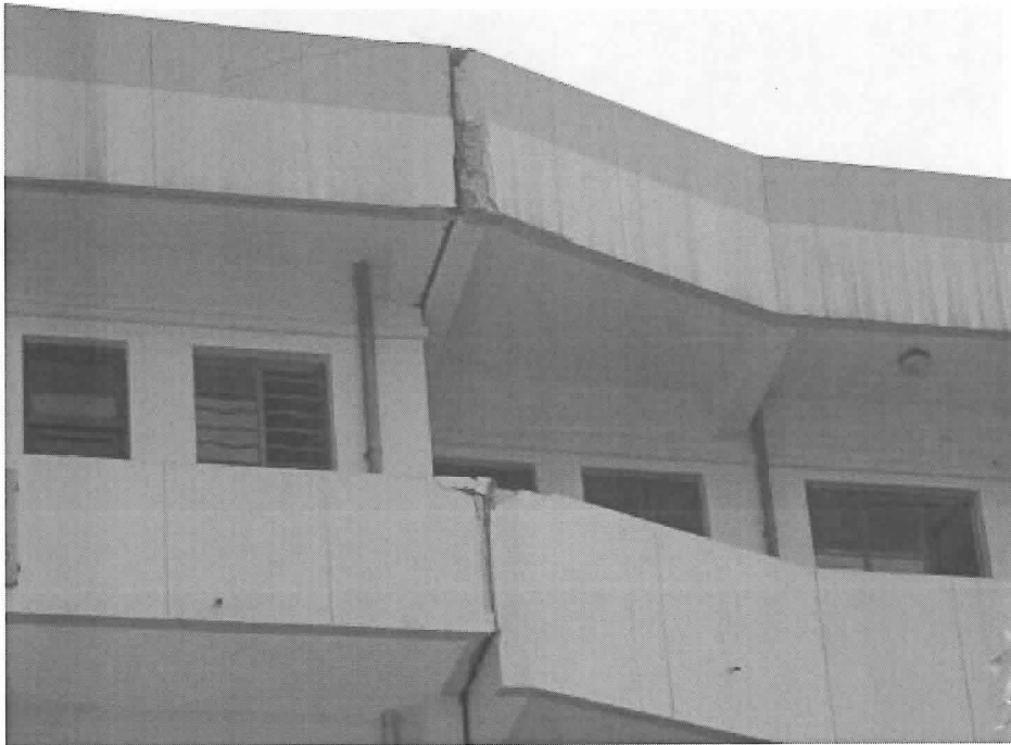
Fig.67. Damage of seismic joint
