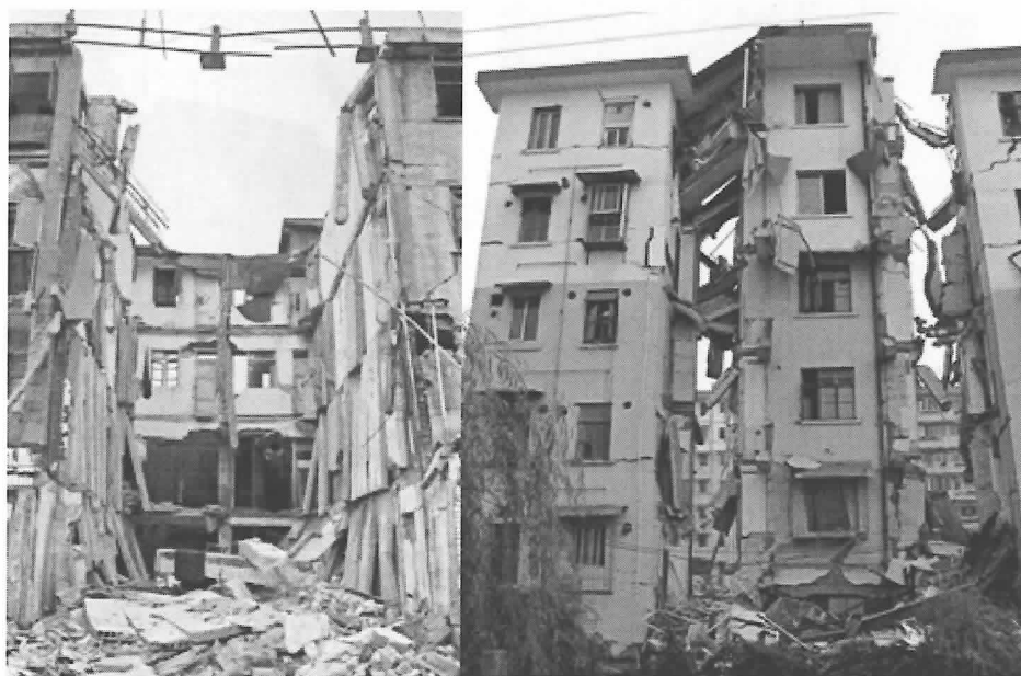
Fig.27. Destruction of masonry structure in Hanwang
