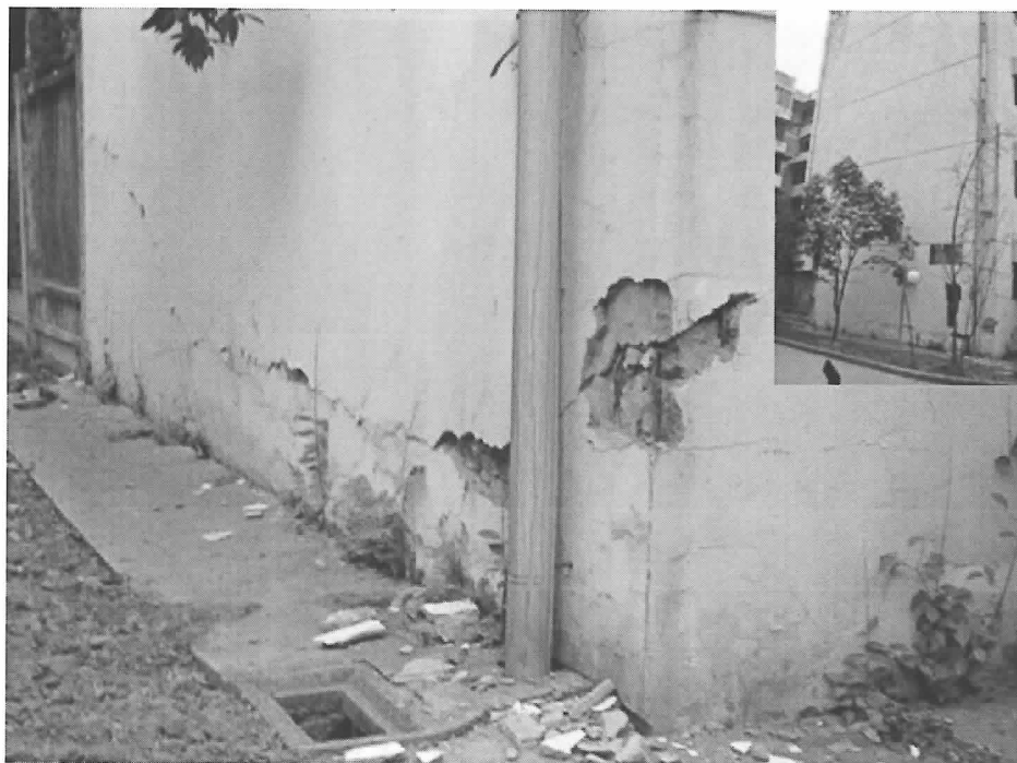
Fig.23. Level cracks in the masonry structure at the bottom in Mianzhu
