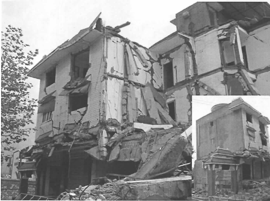
Fig.31. A damage of masonry structure with bottom frame in Hanwang
