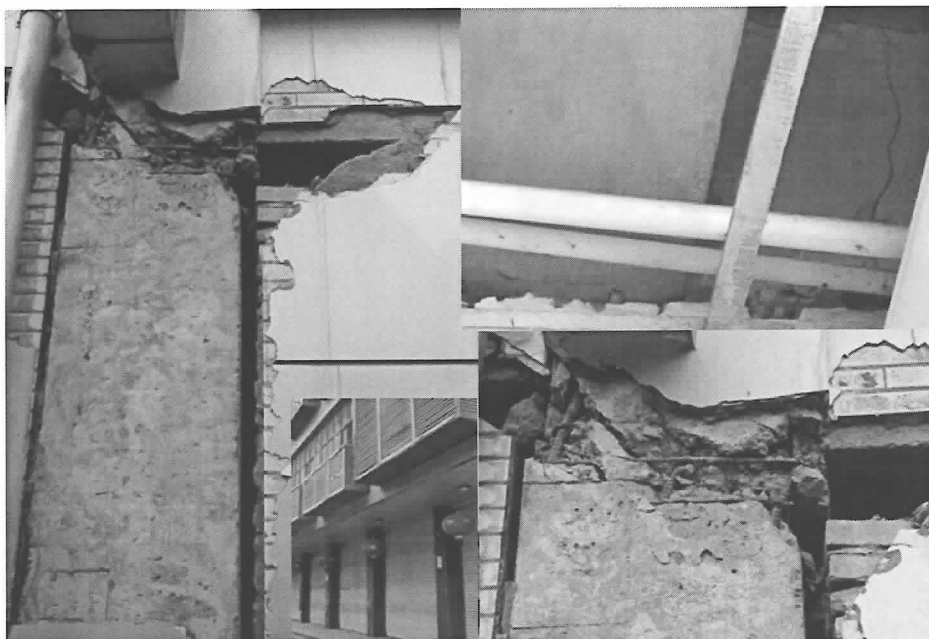
Fig.36. Beam and column damage of frame structure in Mianzhu
