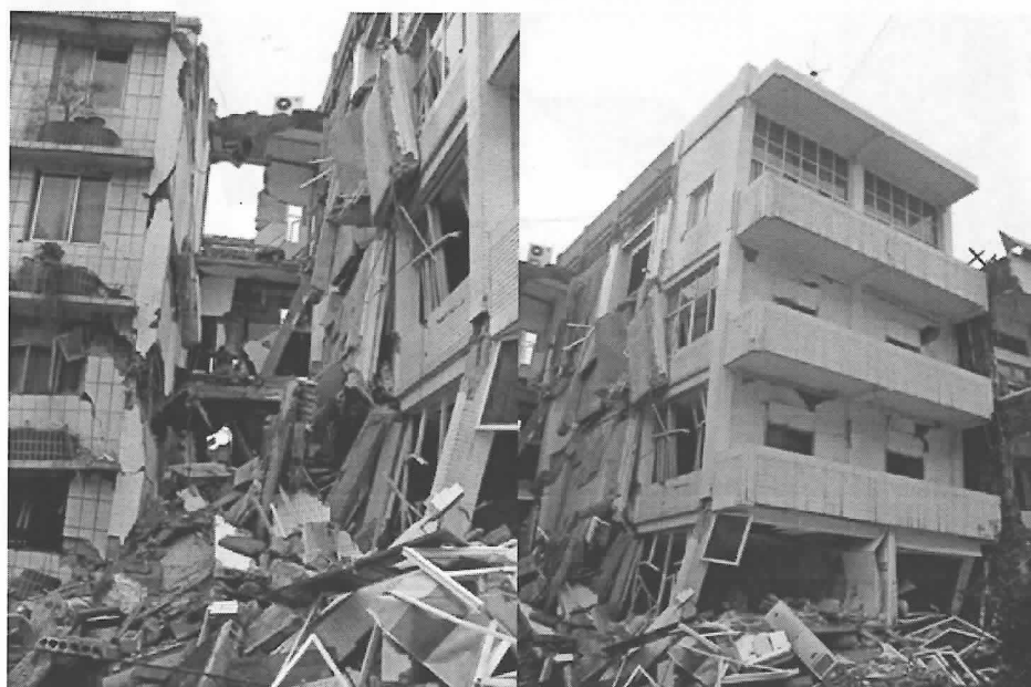
Fig.38. Damage of frame structure with precast slab floor in Mianzhu
