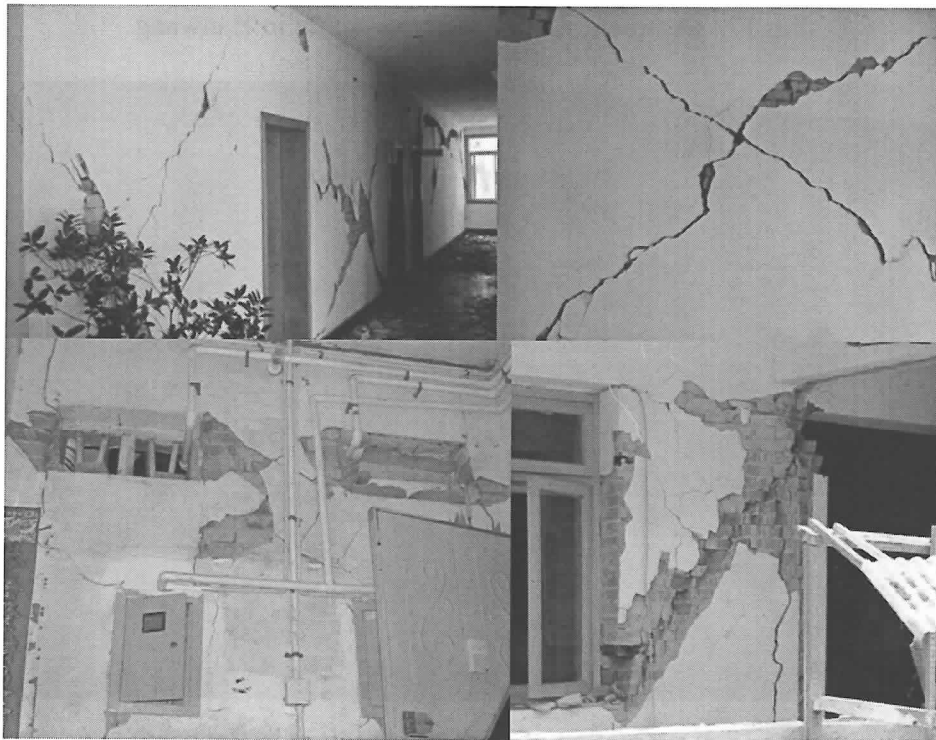
Fig.20. Destruction of the wall forms in Mianzhu
