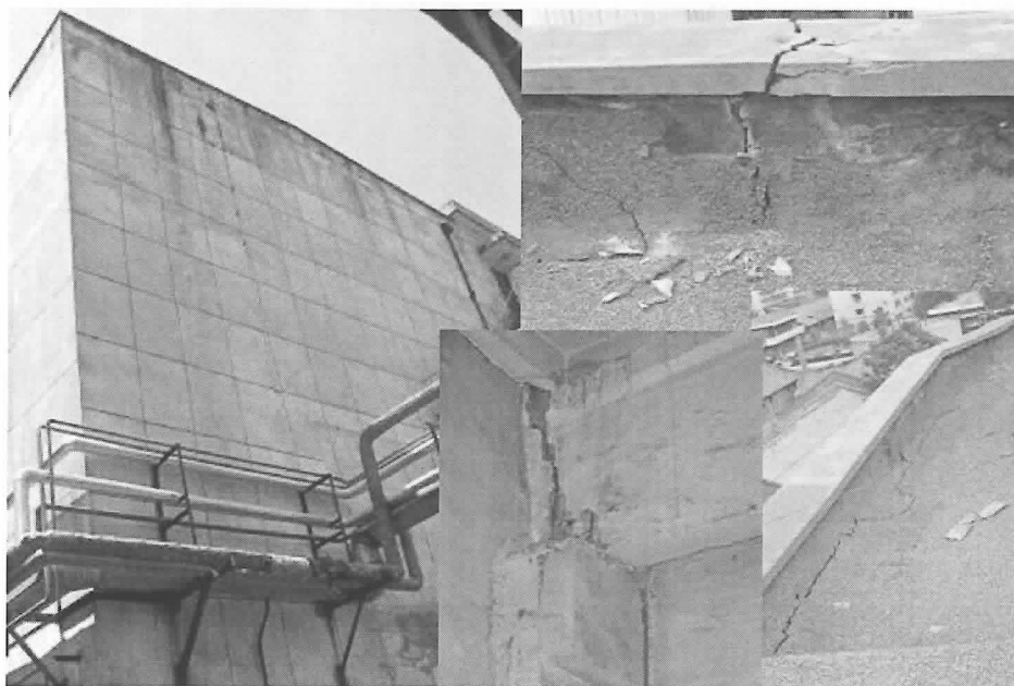
Fig.88. Vertical cracks in the gable and roof beam damage of boiler room workshop
