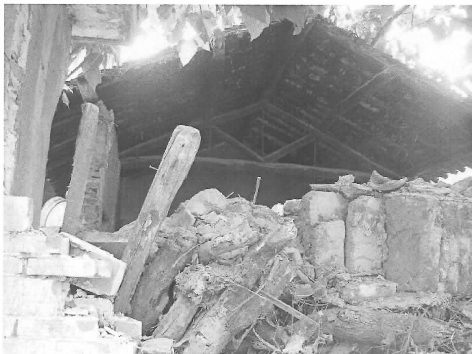
Fig.73. Collapsed adobe house
