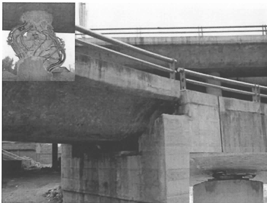
Fig.16. Destruction of roads flyover overpass in Mianyang
