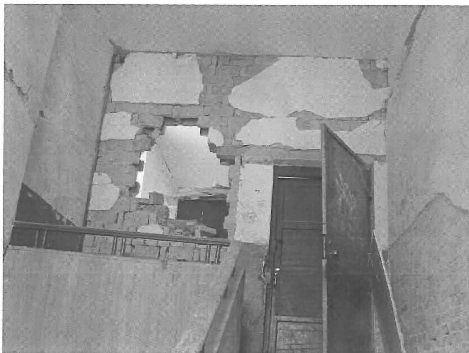
Fig.61. Damage of filled wall
