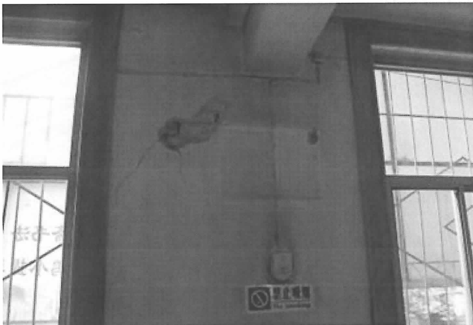
Fig.78. Bearing wall damage under beam
